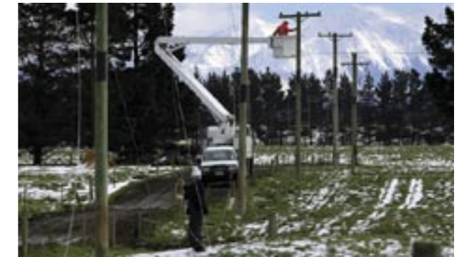
Above: Workmen replace lines following the September 2005 snow storm.
