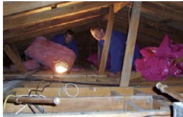
Above: CEA employees installing insulation.
