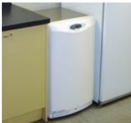
A WhisperGen unit installed.
