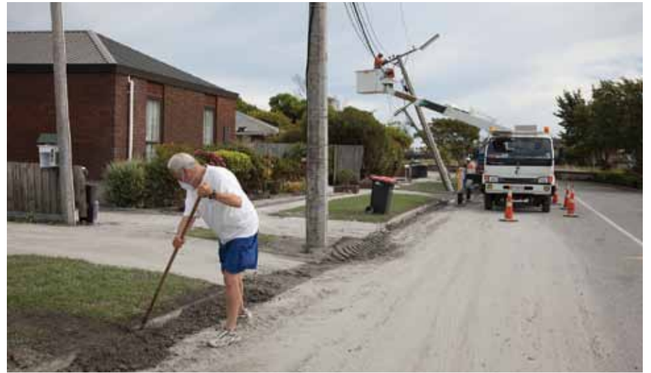
Working alongside residents to repair power lines.
