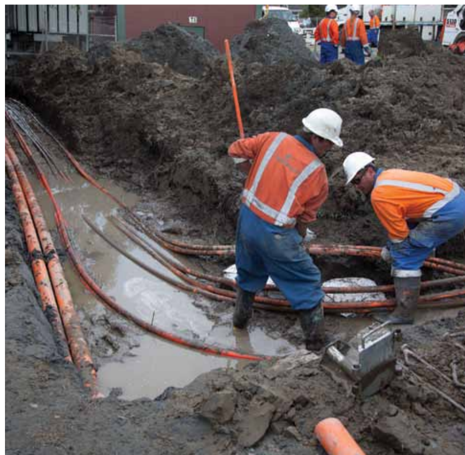
Repair crews replace damaged 11kV cables on Bexley Road.
