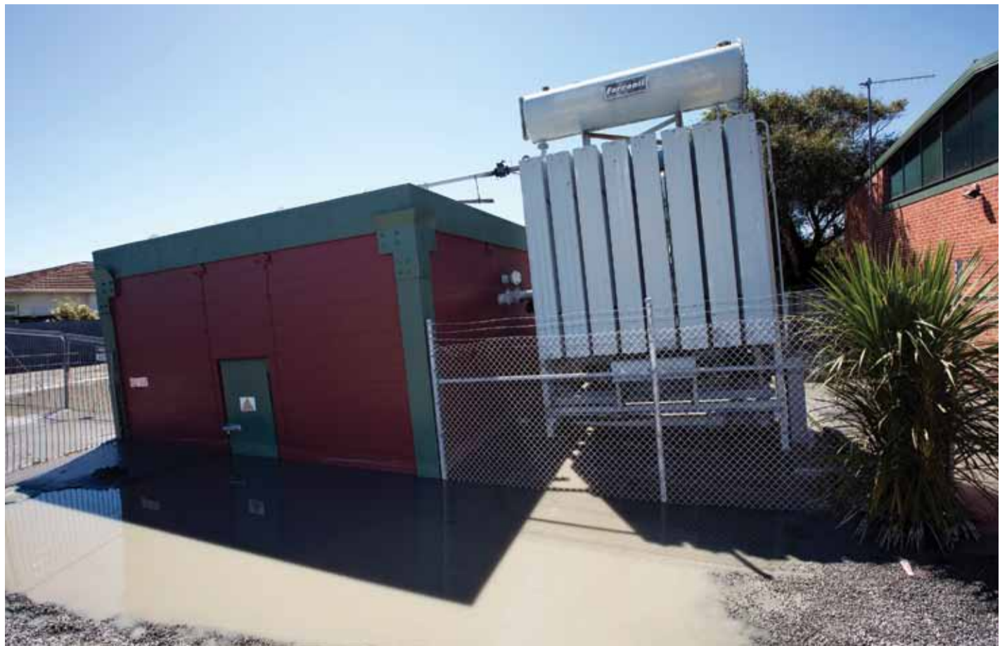
Above: Part of the Pages Road substation which sunk two metres into the ground. Left: Cleaning out the damaged substation.
