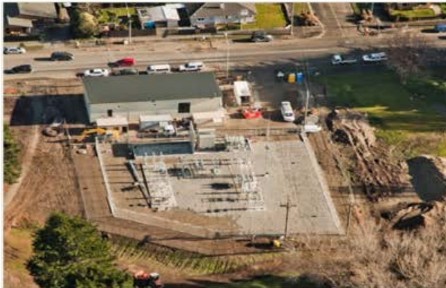
Figure 28: Replacement Zone Substation
