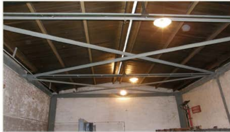
Figure 27: Substation Strengthening - Steel Framing
