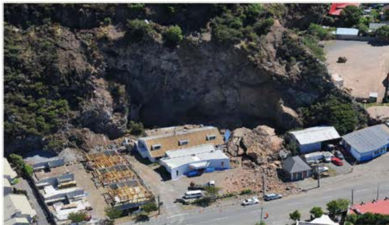
Figure 20: Substation Damage from Bolder - Wakefield Avenue
