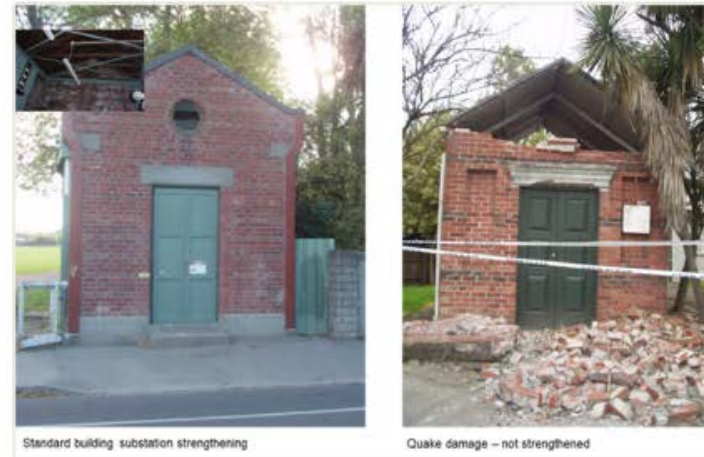
Figure 19: Substation Damage Comparison
